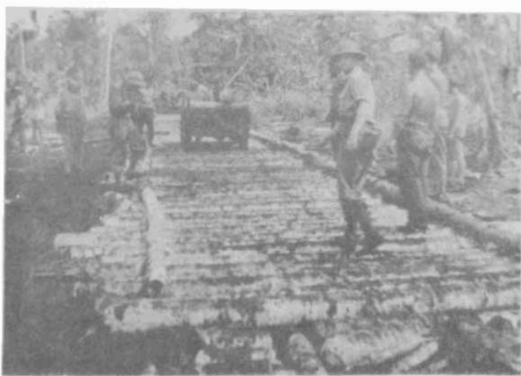
. . . a completed section.
